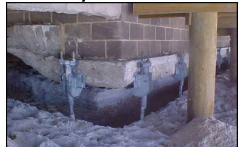
Exterior Footing Supported by Helical Piers
