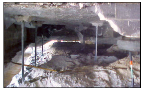
Close up of Area A: Concrete Slab Supported by Helical Piers
