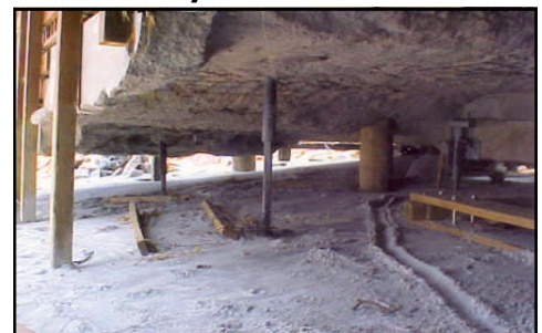
Slab & Grade Beam Supported by Helical Piers
