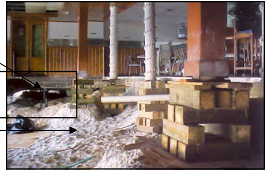
Close up of Area A: Concrete Slab Supported by Helical Piers
